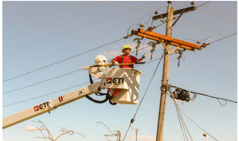
Above: Hillsboro crew member Jason Plett, reestablishing electric service.
