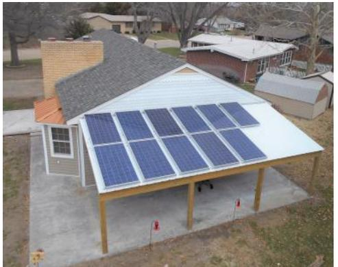
A new 3.8 kW rooftop system installed in Ellinwood utilizing the City's interconnection ordinance.
