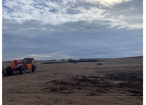
Progress photo at site for Kingman/Cunningham substation
